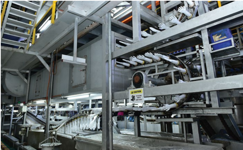
Glove manufacturing facility at JREMT
